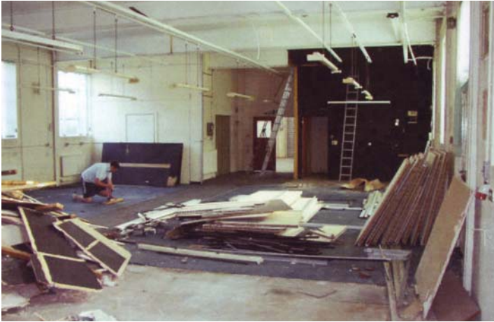
The derelict building on its way to transformation
